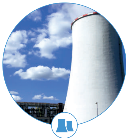
ELECTRICAL POWER GENERATION
