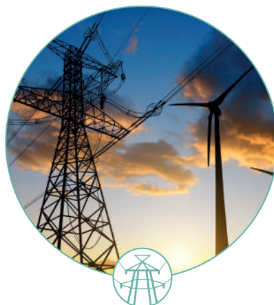
ELECTRICAL POWER TRANSMISSION AND DISTRIBUTION
