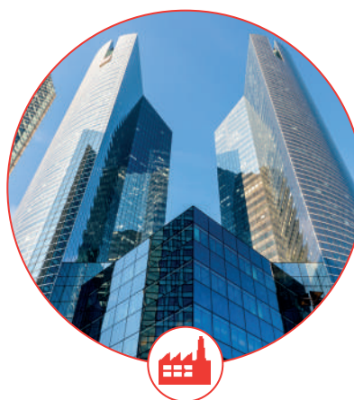
INDUSTRY AND TERTIARY BUILDINGS
